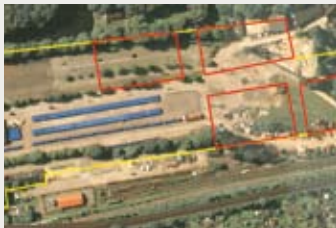
Bird's eye view of the Alte Wöhr construction site
